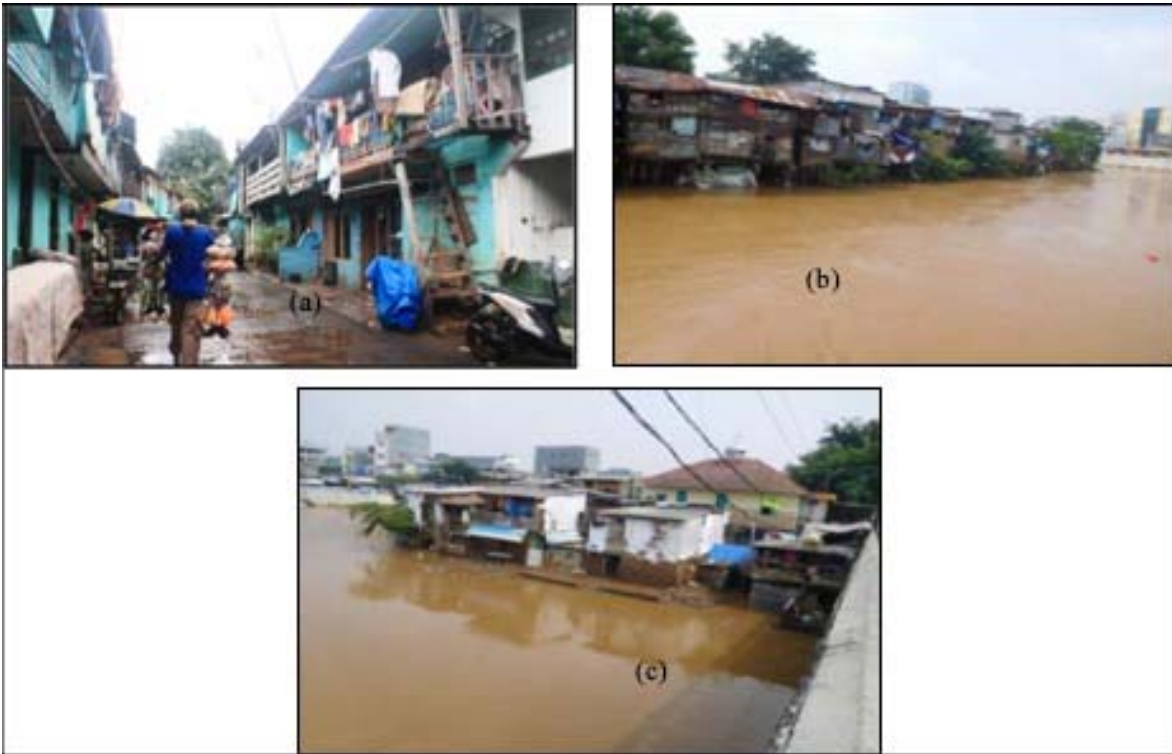
Figure 3. 4.(a) Housing conditions, (b) riverbank settlements, and (c) post-flood inundation damage
