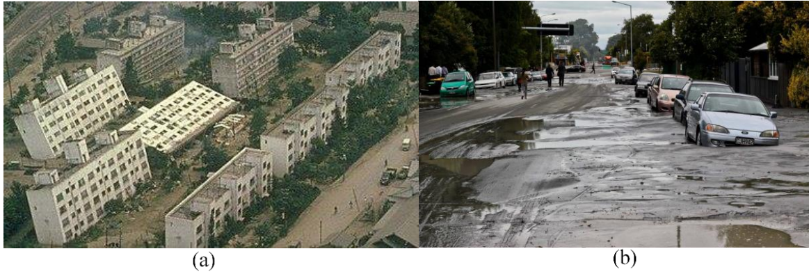
Figure 2.5 (a) Tilting of buildings due to Niigata Earthquake (1964), (b) Extensive damage of the road in Christchurch caused by earthquake (2011)
